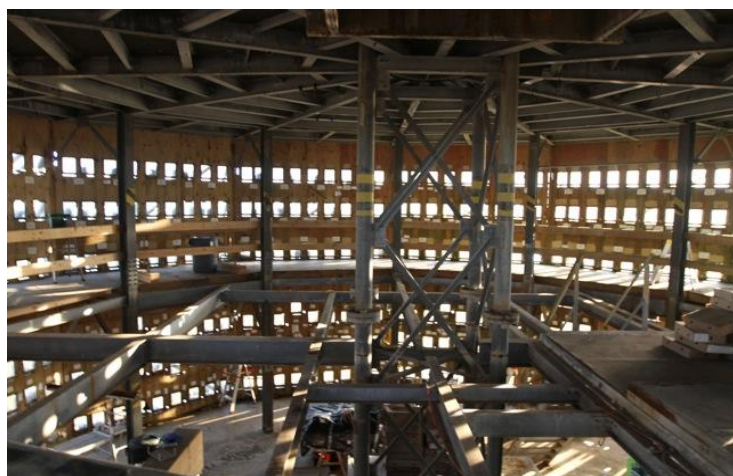
View of the inside of the Middleton Island tower. Behind each of the one-way mirrors is a kittiwake nesting site. (Photo by M. Johns)
